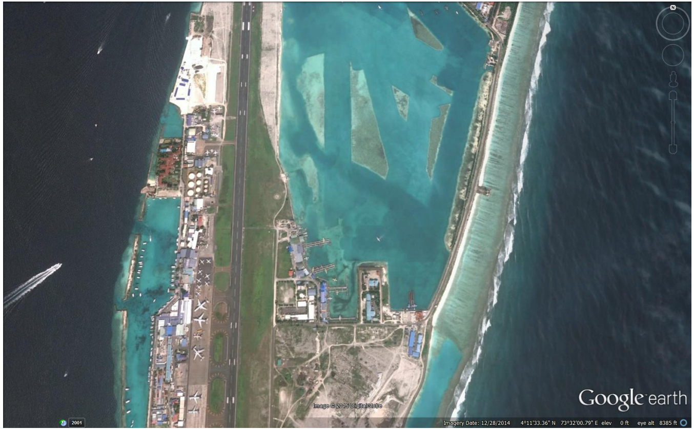
Water Aerodrome, Ibrahim Nasir International Airport
